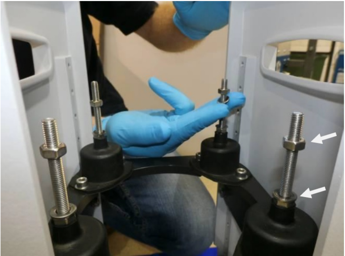
Figure 5.8: Removing the upper nuts from the anti-vibration (AV) mounts
